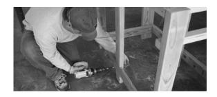
O9 The inside edge of the top front stretcher (J) should fall across the center of the top of the front middle leg (E), leaving about 3/4" for both the top front stretcher and middle upper stretcher (G) to attach to the leg. Place middle upper stretcher on top of the back and front middle legs (E) and attach with 3" screws. Drive 3" screws through the front of the top front stretcher and into the middle upper stretcher as well.
