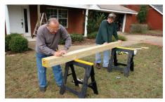
**3.** Measure new column (be sure to account for the added height of the plinth) and cut to the same length as the old.
